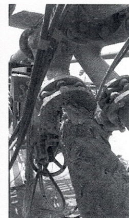
Leakage valve body due to ash abrasion
