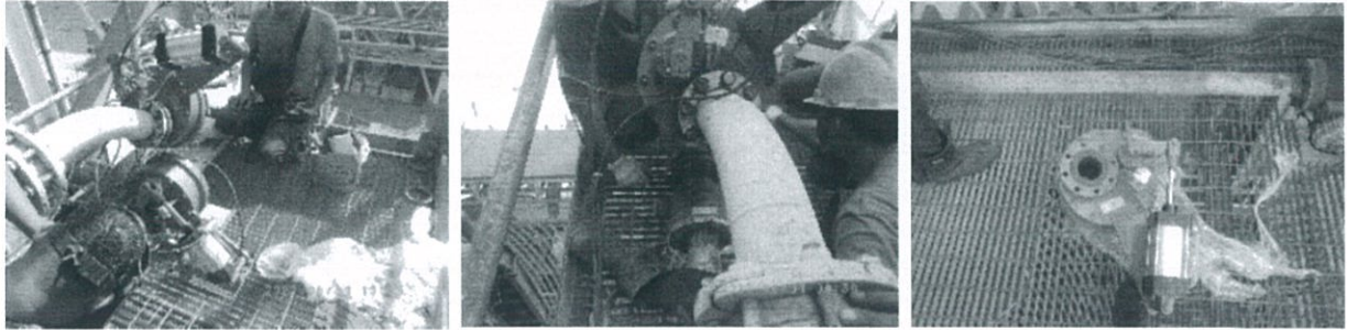
Unit 4 RDDV installation
