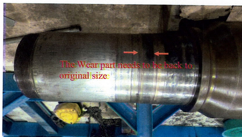
IDF Main Shaft Condition after dismantled main bearing
