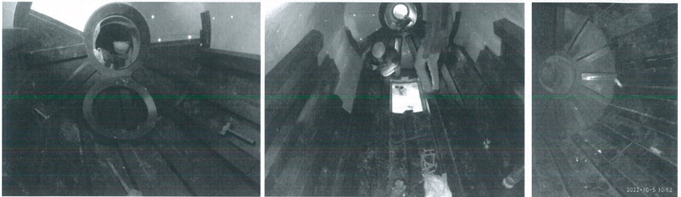
Install new rubber lining
