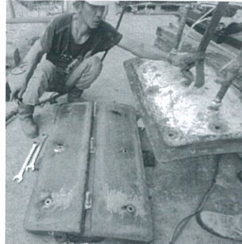
Rubber lining installation
