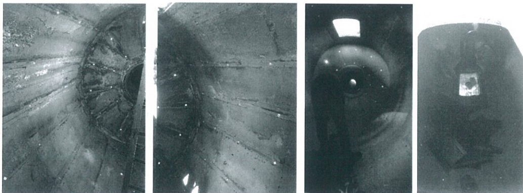
Cleaning & painting inside drum
