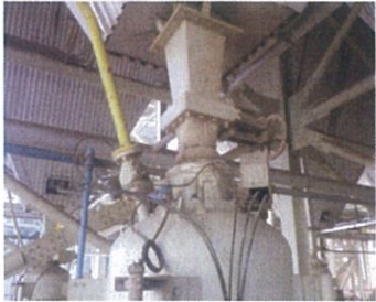
DN200 Dome Assembly: 1. Eco,AH in & out pump 2. ESP Field 1~ 4 pump
