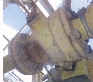
DN80 Dome Assembly: 1. Eco & AH in LSV 2. AH out LSV 3. ESP Field 3&4
