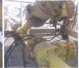
DN80 Dome Assembly: 1. Eco & AH in LSV 2. AH out LSV 3. ESP Field 3&4
