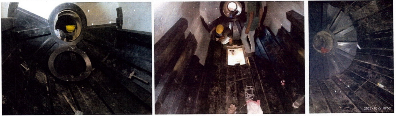
Install new rubber lining
