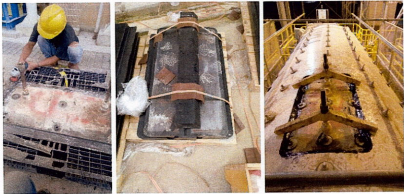
Fabricating and install manhole
