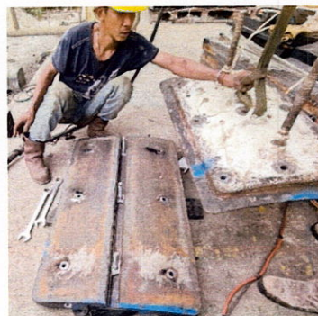
Rubber lining installation
