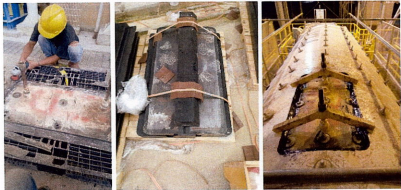
Fabricating and install manhole
