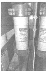
A480R12R-1, 2400V/4800V, 50/60HZ,FERRAZ SHAWMUT
