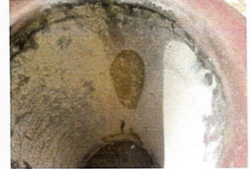
eroded plate at inlet chute
