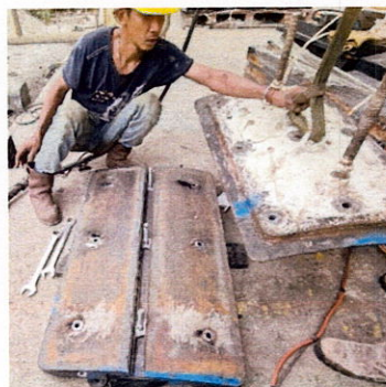
Rubber lining installation
