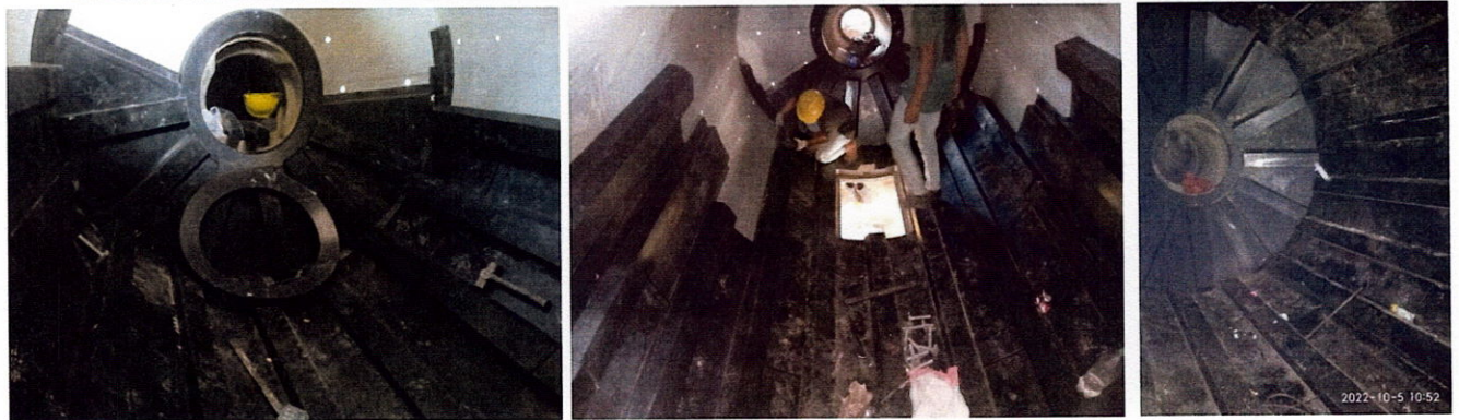
Install new rubber lining
