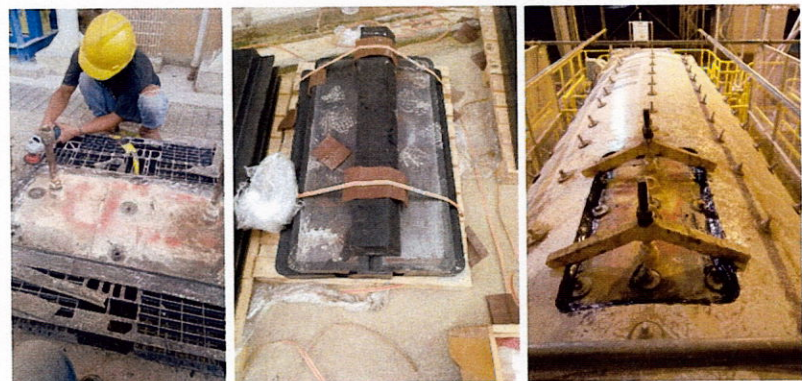
Fabricating and install manhole
